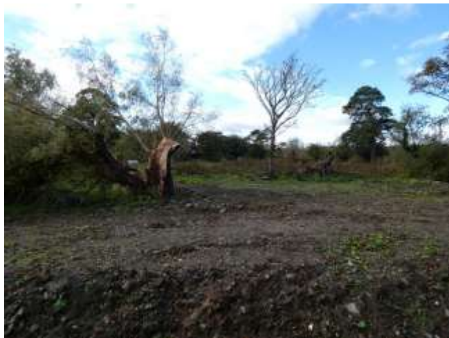
Figure 10.9: Cleared ground at Site Compound 1 behind the Petrol Station on the Dublin Road with Willow and Pine.
