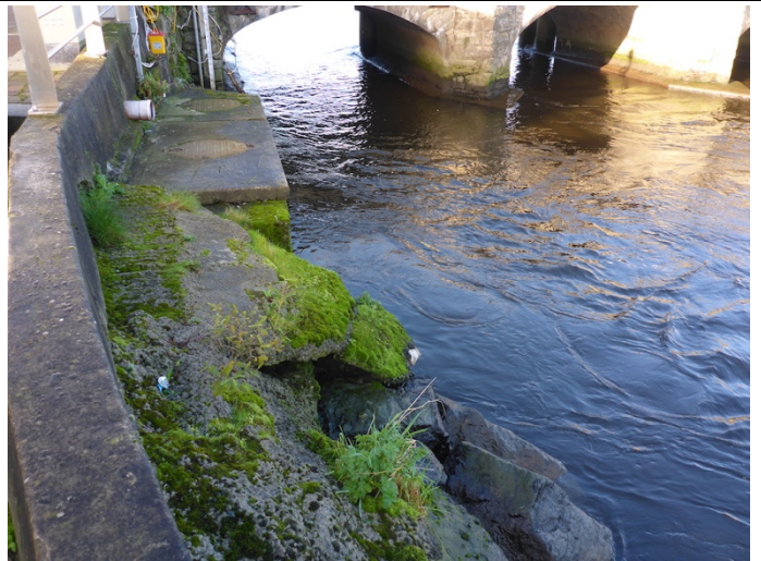
Photograph 3.8. Concrete wall and stonework at the edge of the river, downstream of the bridge. Bryophytes locally frequent and dominated by urban species of walls and disturbed ground. S bank of the river.
