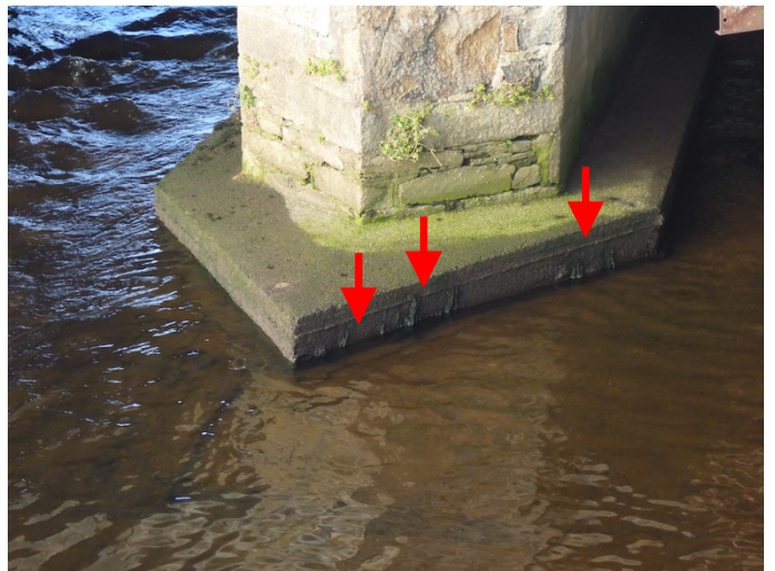
Photograph 3.6. Stonework on bridge arches (below high tide) has little/ no bryophyte cover. Red arrows show the small amount of aquatic moss Fontinalis antipyretica . E side of bridge.
