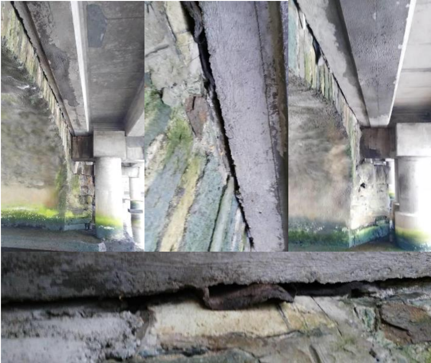
Bridge crevices under which bat droppings indicate use of the bridge by roosting bats T2530673188
