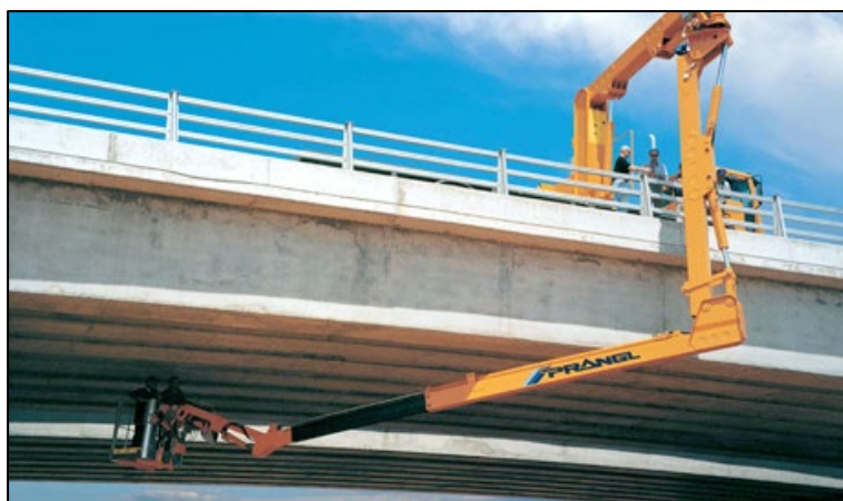
Photograph 5 - Aerial Mobile Platform
