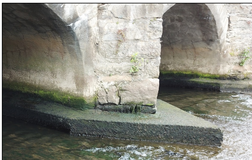
Photograph 3 – Masonry Joint Defects
