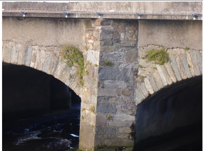
Photograph 3.5. Stonework on bridge arches (above high tide) has little/ no bryophyte cover. E side of bridge.
