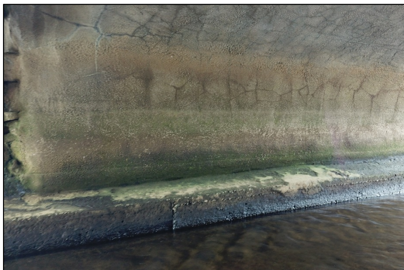
Photograph 2 – Cracking of Bridge Soffit Repairs
