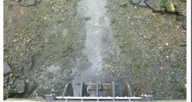
Plate 12: Sewage fungus at flap valve on the South Quay
